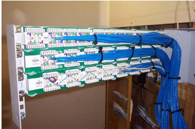
**Step 6: Test the data jack and patch panel terminations with a basic cable tester (optional)**
